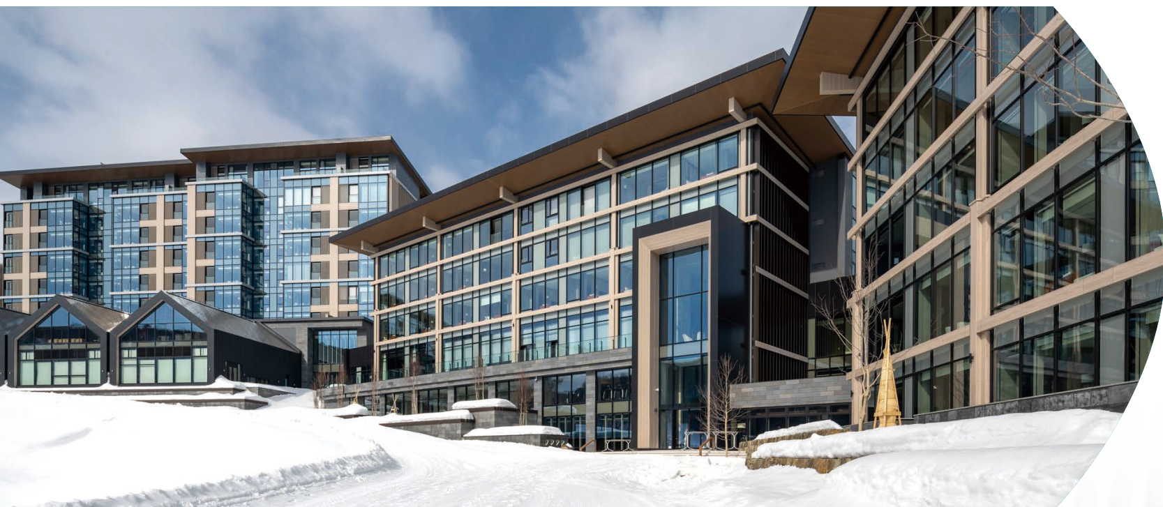
Park Hyatt Niseko Hanazono Residences and Park Hyatt Niseko Hanazono in Japan
